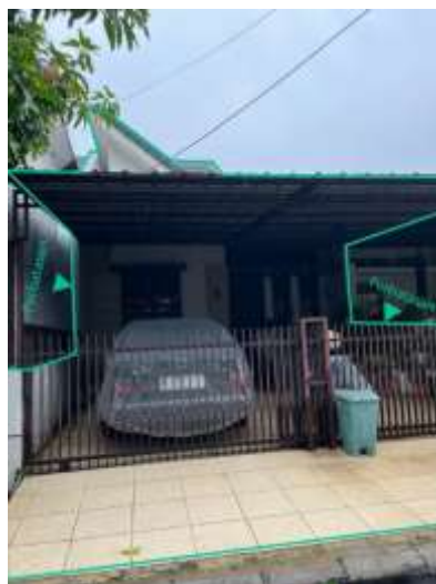
Figure 6. Condition of a House Directly Bordered by Buildings on Both Sides
