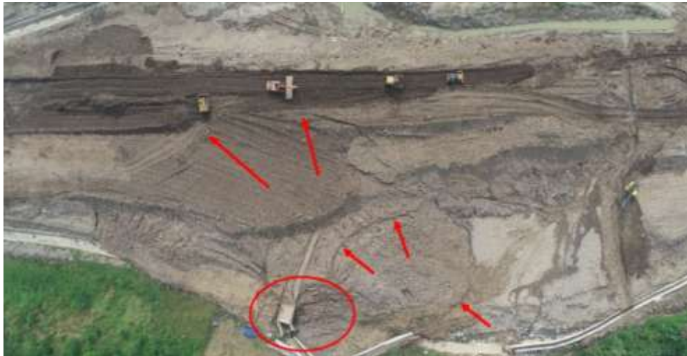
Figure 3 Cracks in STA 40+200
