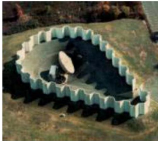
Figure 7. Construction of a protective shield on the FSS
