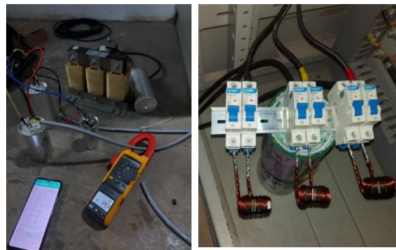
Figure 14. Fifth-order single tuned LC passive filter assembly
