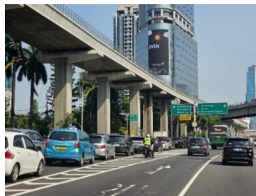
Figure 5 Tegal Parang Off Ramp Situation (KM 5+000 A)
