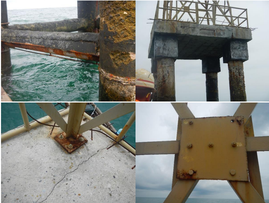
Figure 2. Damage to Gosong Pasir Lighthouse Before Collapse
