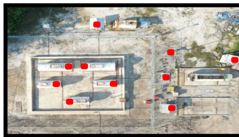
Figure 3 The red dot is the location of the sensor installation in the fuel storage area
