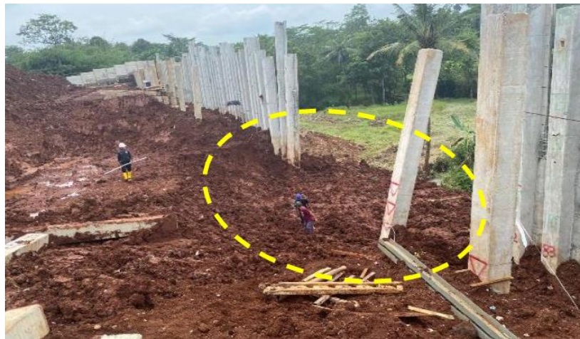
Figure 5. Condition of Landslide Soil and Completed Reinforcement
